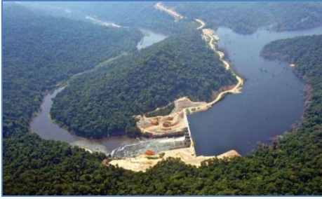
Nam Theun 2 hydropower dam on the Mekong River tributary in Lao PDR
